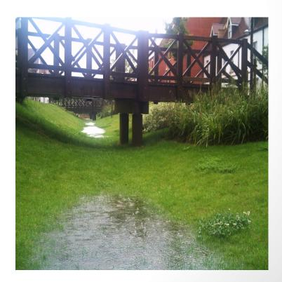
Network of swales and green space but uses gullies before swales forcing a greater depth of swale
