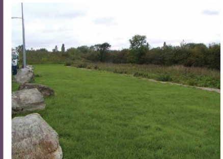
Figure 15.1 Filter strip at motorway services draining to filter drain, Hopwood (courtesy Ilman Young)
