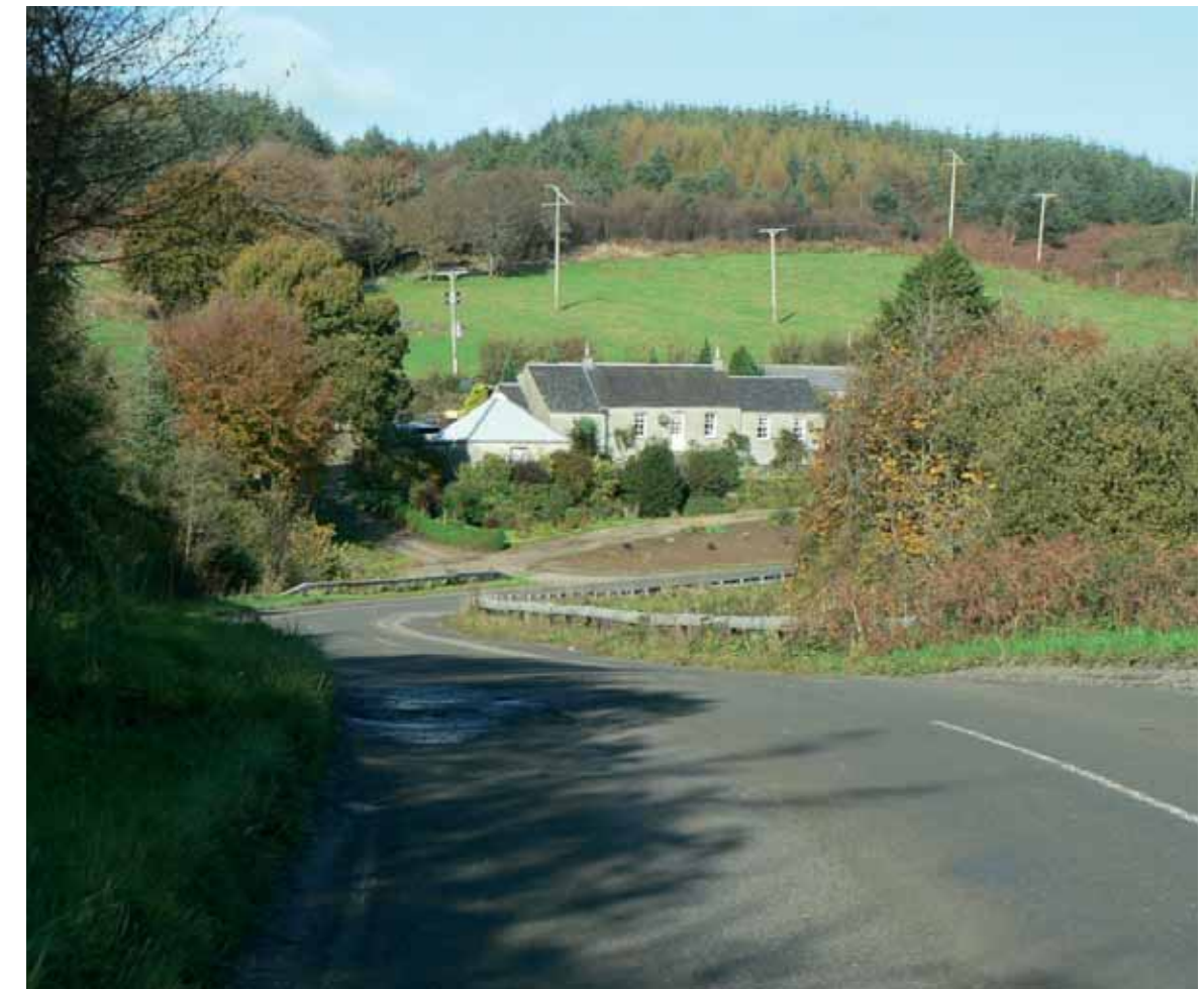
SK19 - Looking north into ROA towards Bunlarie
