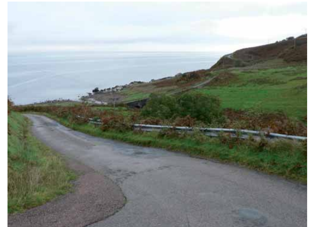
SK15 - View east to Corphin Bridge
