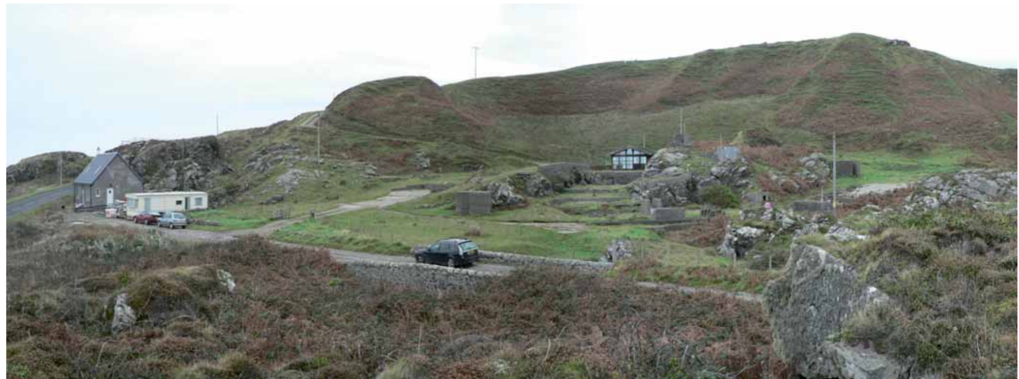
SK4 - Dun Putechantuy indicating existing buildings
