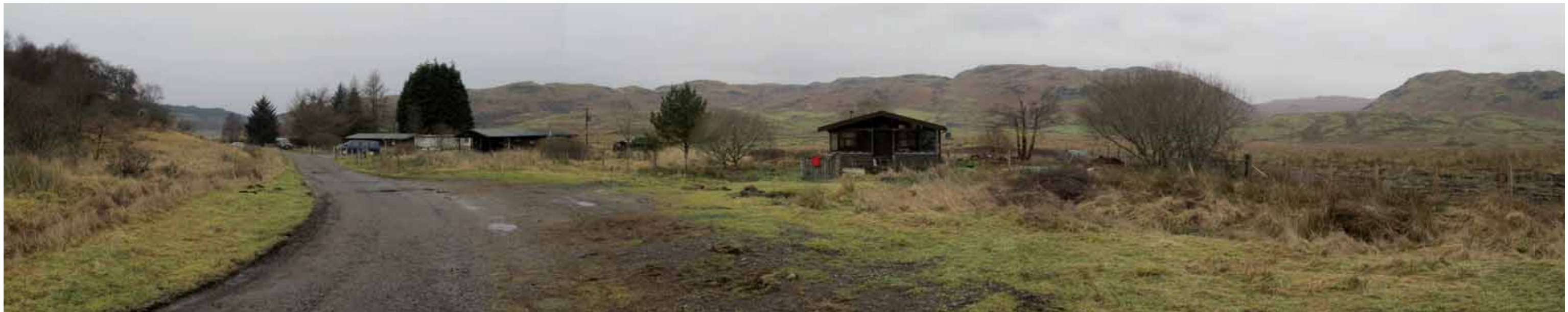
LN77- Holiday Chalets along the southern boundary of the site
