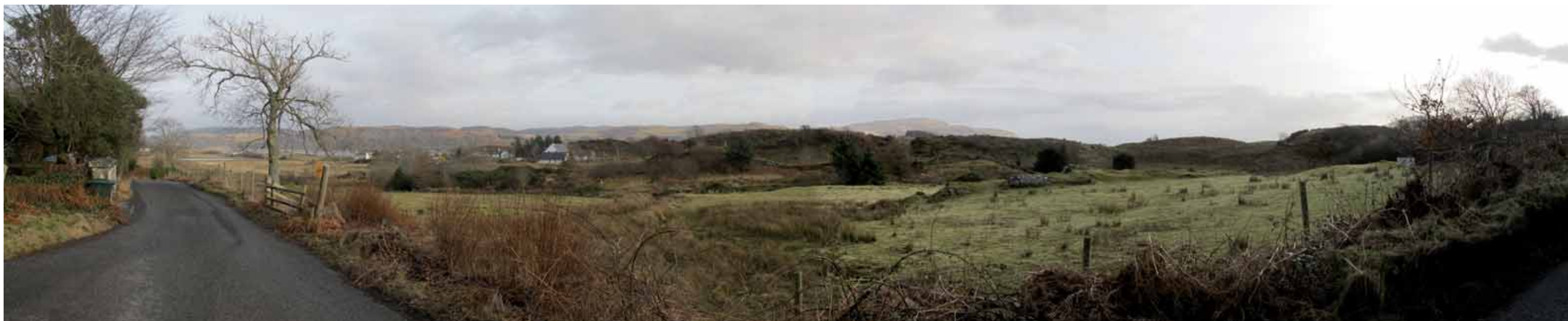
LN62- View west of the B844 in the northern part of the site
