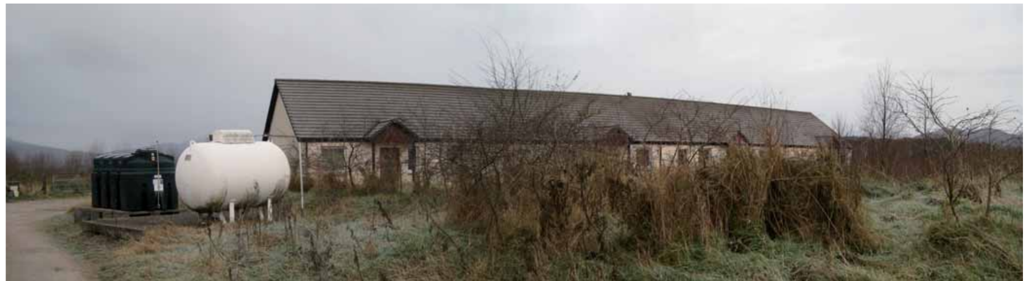
LN27 - Existing development at the northern end of the site
