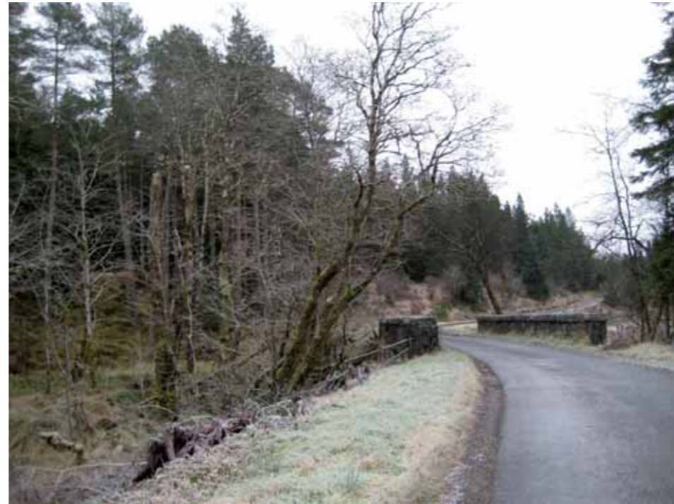
LN24- View into ROA over bridge
