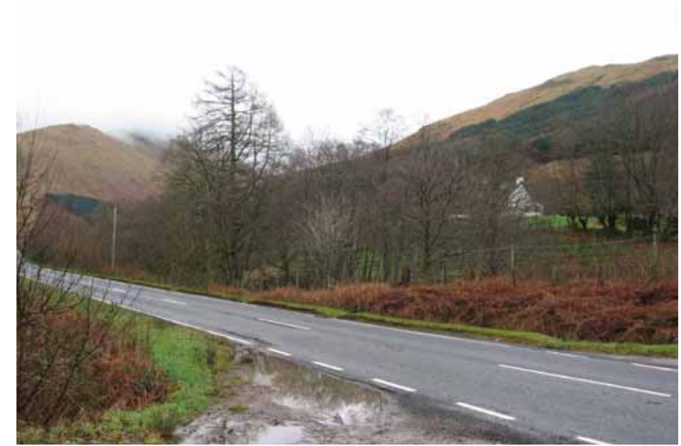
CB51 - Looking towards Croft Kennels
