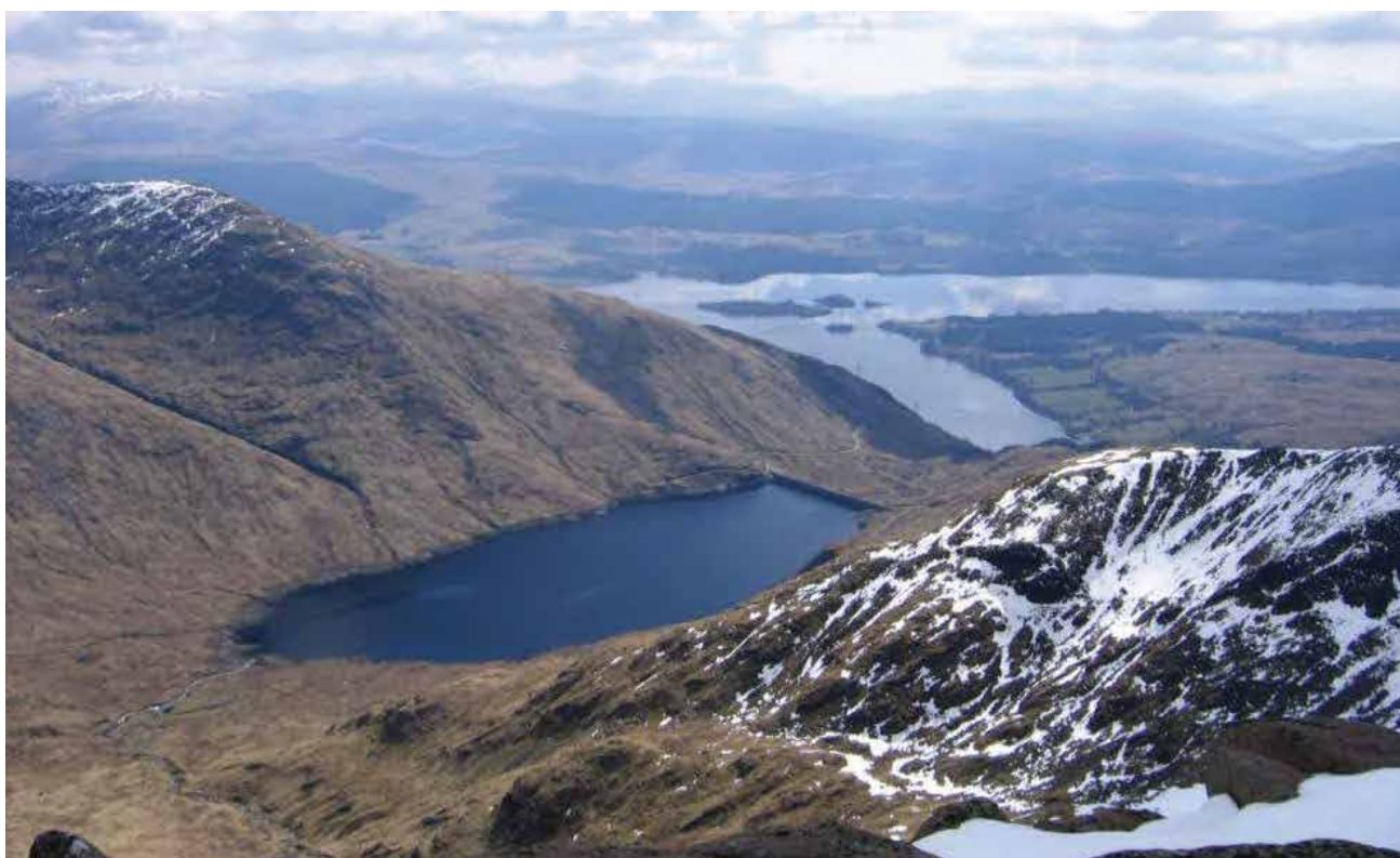
Photo: Cruachan Reservoir and Dam
