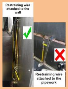
Connecting and disconnecting plugin gas connections on appliances when moving for cleaning, or changing LPG cylinders or hoses can be carried out by you but you must be competent.
