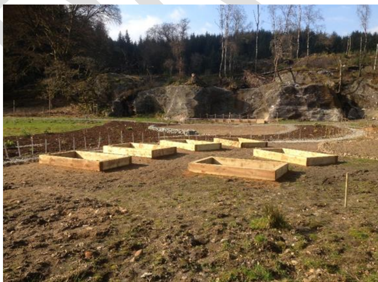
Lochgilphead Community Growing Space- construction phase.
