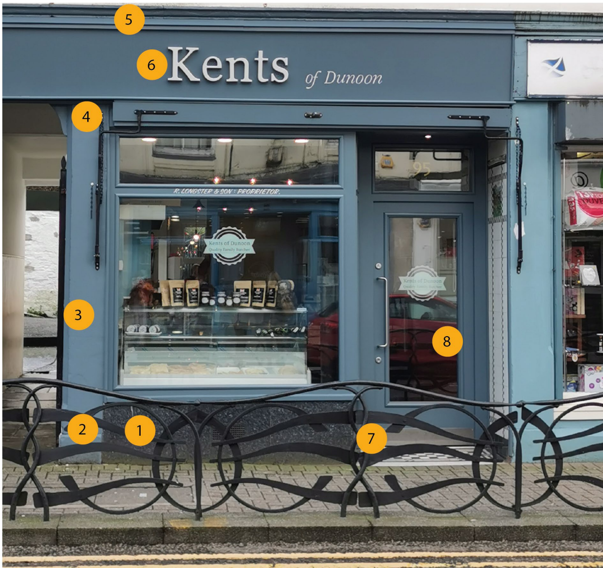
(1) Stallriser, (2) plinth, (3) pilaster, (4) area for console bracket, (5) cornice, (6) fascia, (7) recessed entrance, often enclosed by timber panelled storm doors (8) inner glazed doors
