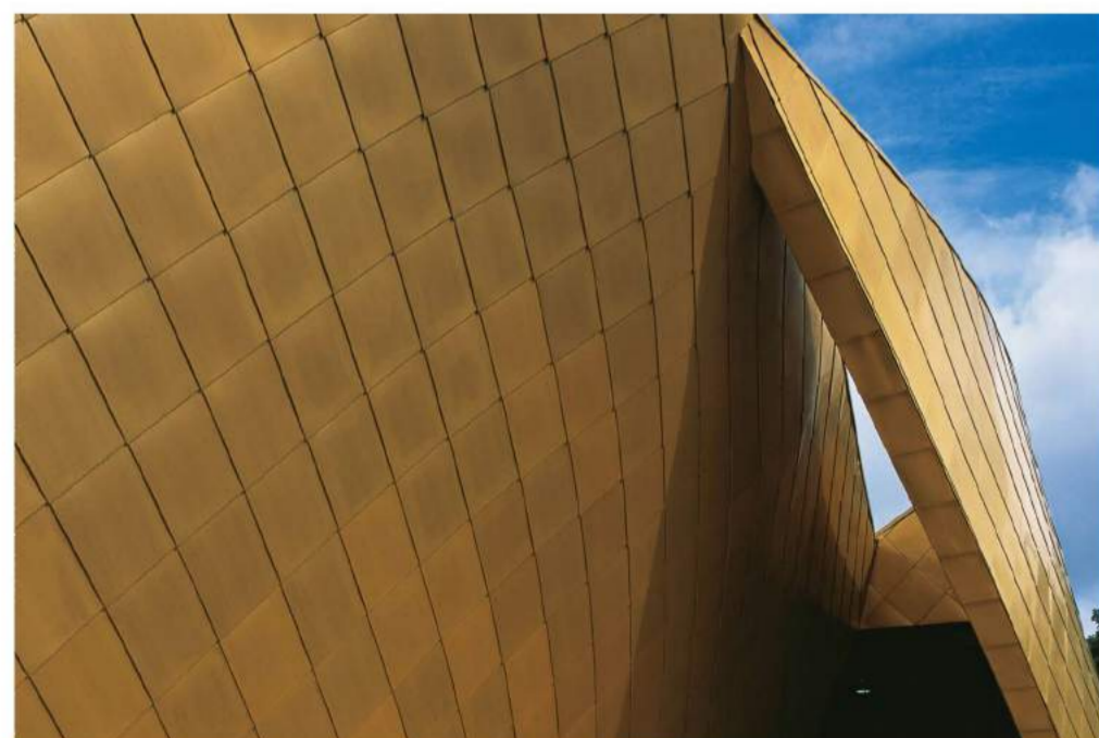
COLOURED ZINC CLADDING WRAPS AROUND FIRST FLOOR
