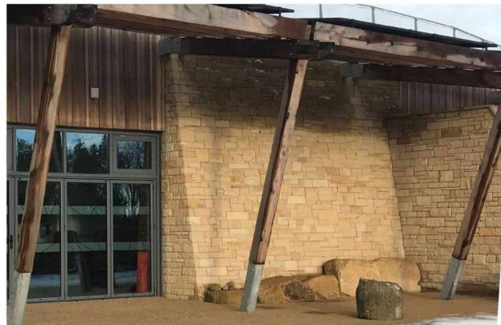
ANGLED BUTRESS WALL TO BASE OF BUILDING
