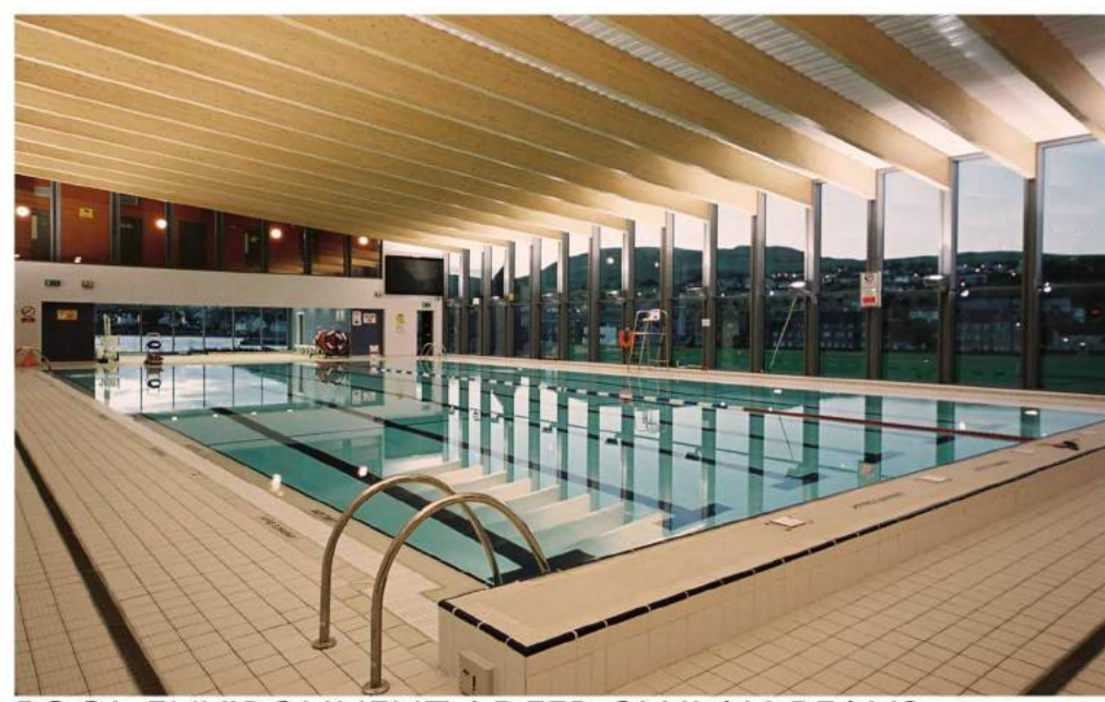
POOL ENVIRONMENT / DEEP GLULAM BEAMS
