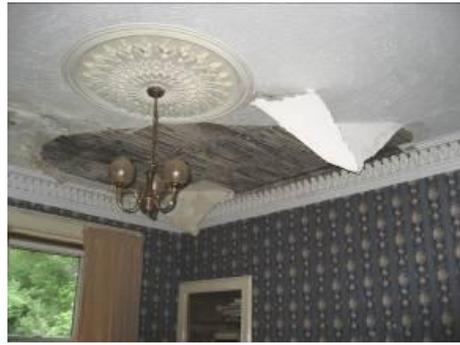
Water ingress causes ceiling collapse
