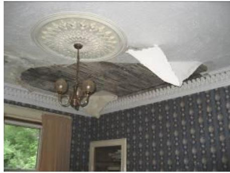
Water ingress causes ceiling collapse
