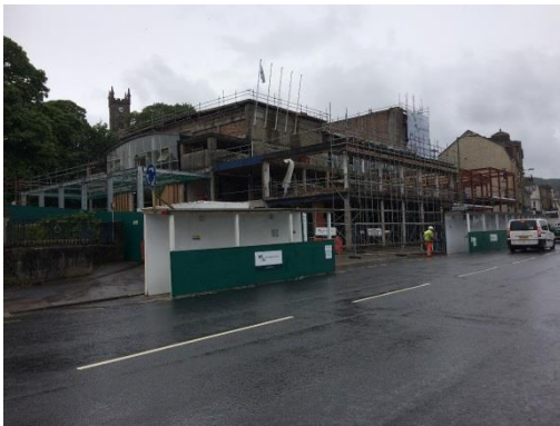
Southern and Western Elevations
