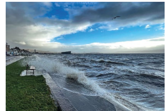
Seawater breaking over the Promenade
