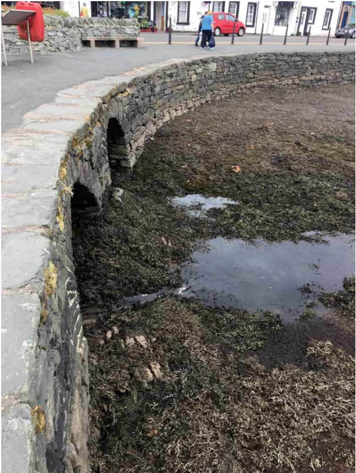
Photograph 1: Outfalls into harbour for Back Road and Ileene Road culverts
