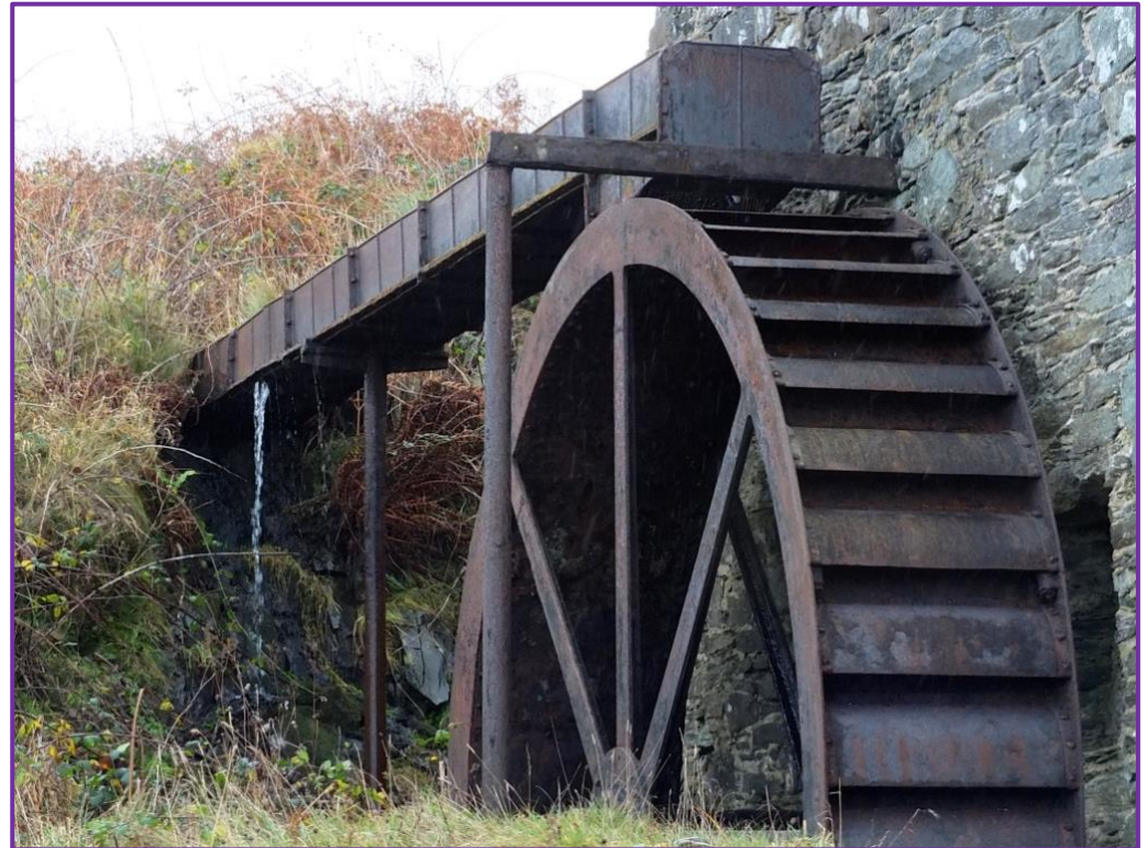
The Ardailly Mill was once powered by the supply from Upper and Mill Lochs.
