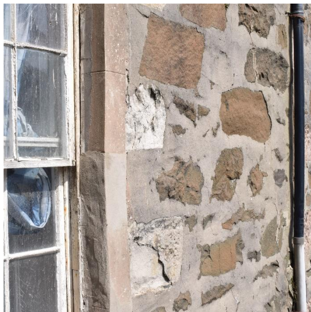
Typical rear rubble stonework – cement pointing and decay of window surround stonework
