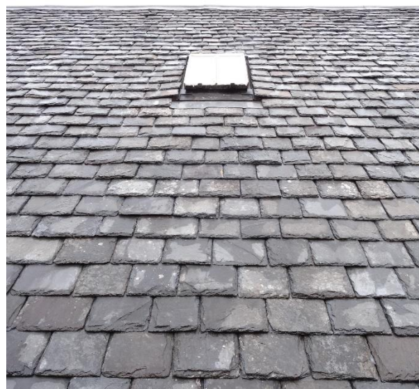
Re-slatted roof using traditional Scottish slate in diminishing courses and random widths at MacQueens of Rothesay Butchers 1-3 Bishop Street.
