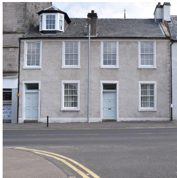
51-53 High Street. A good example of traditional timber sash and case windows and a demonstration of their importance to the overall character of the building. 6 over 6 glazing pattern formed with astragals.
