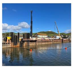
The remaining works are the completion of cope installation, installation of quay furniture (bollards, ladders, fenders), completion of dredging works, site reinstatement. The completion date for the project is 04 October 2025.
