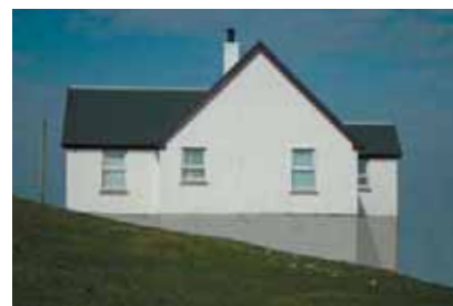
this house is located on a steeply sloping site, so it needs a significant level of underbuilding
