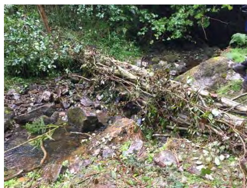
Figure 4-3 Newly constructed woody debris dam in Yorkshire Dales
