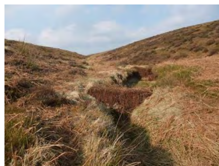
Figure 4-5 Heatherbale ditch blocking
