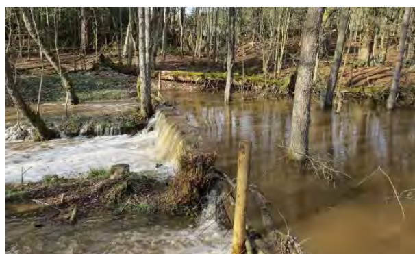
Figure 4-7 in channel engineered leaky barrier (Pickering)
