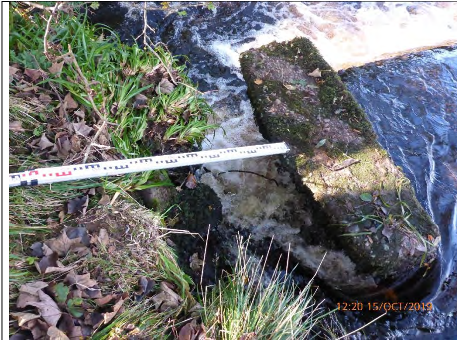
Figure 3: By-pass channel which has started to form on the left side of the weir as the flow cuts around it.
