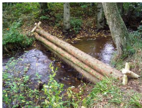
Figure 4-4 Engineered Leaky Barrier
