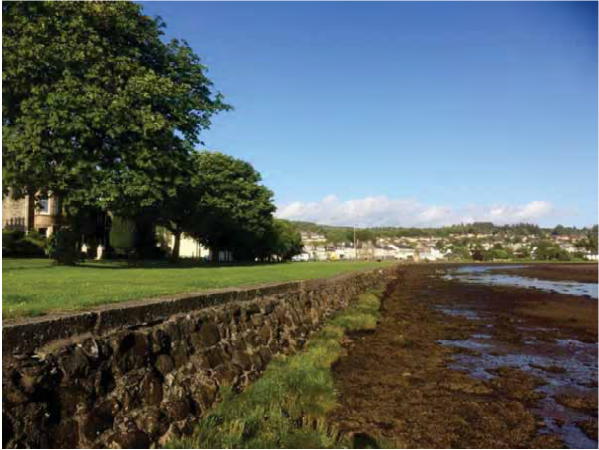
Photograph 8: tidal defences along Front Green
