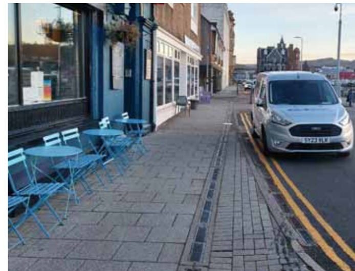
Pedestrian route leading south from Corran Esplanade. The width of footway is reduced by restaurants' furniture
