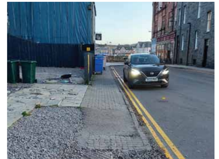
Pedestrian route looking south across from the Oban North Pier. The footway surface remains poor quality
