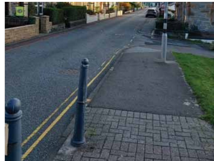
Pedestrian route leading south from A85. Single footway on the west side of Dunollie Road, with uneven and poor quality surface
