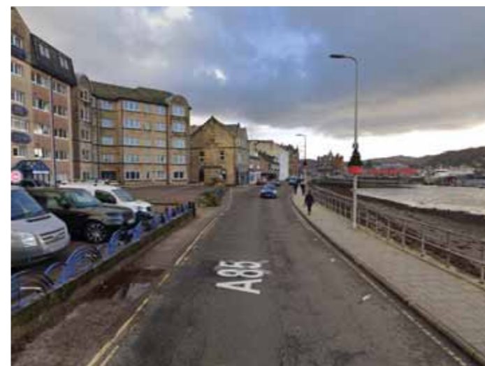
Image 3 | View south on Corran Esplanade adjacent to the Great Western Hotel showing missing footway
