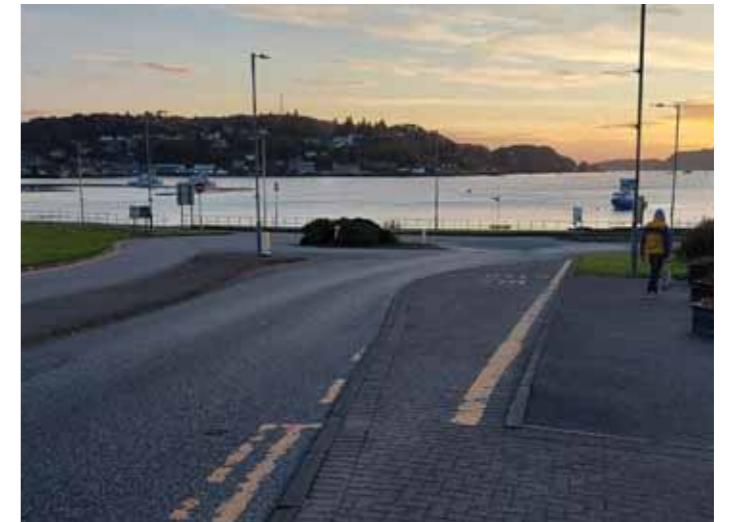
Pedestrian route along A85 linking Dunollie Road to Corran Esplanade. The one sided footway adding difficulty for pedestrian crossing
