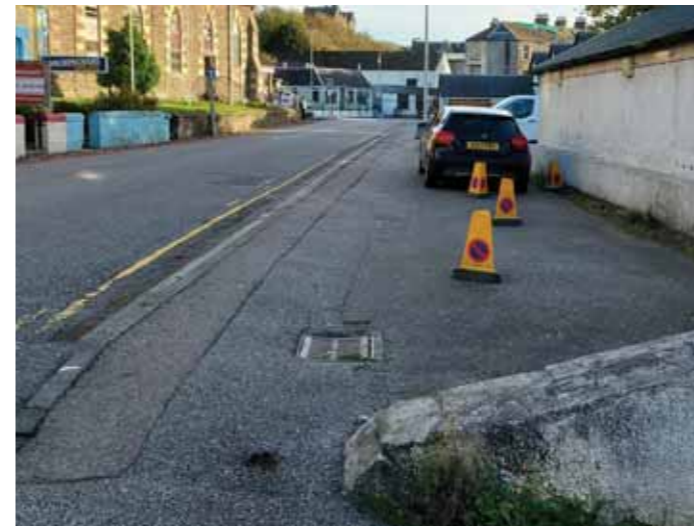
Image 2 | Image shows informal/non-standard parking arrangement on Dunollie Road adjacent to Farm Foods
