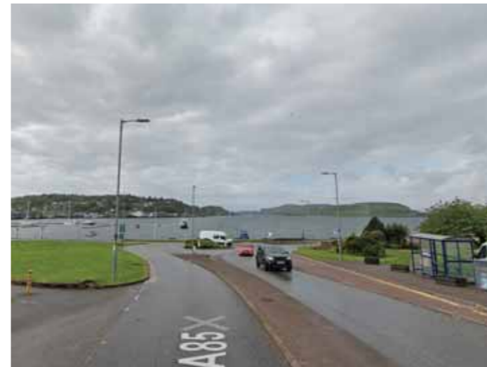
Image 2 | Image showing termination of footway to south side of carriageway and pedestrian refuge island with defensive paving
