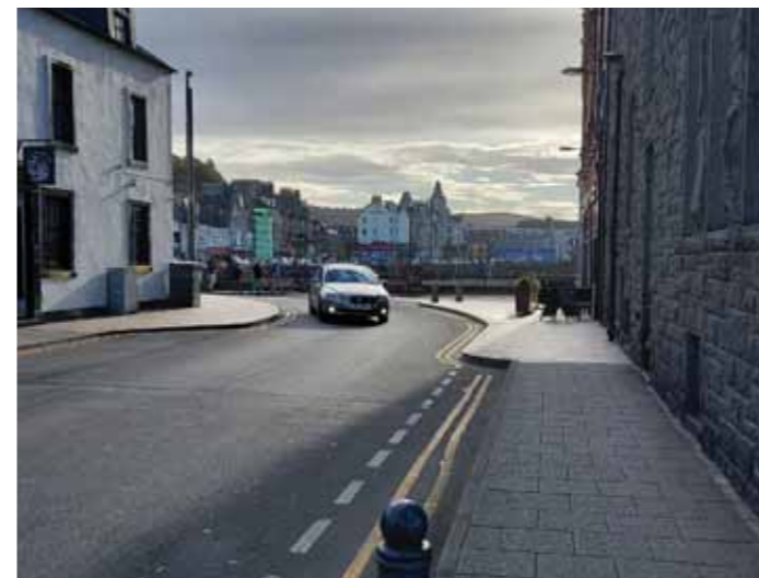
Looking south towards Oban Train Station. The footways contain minor obstructions by bins, feeder pillars, and restaurant's furniture.
