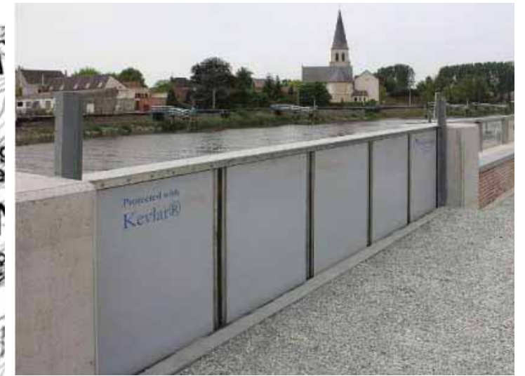
Example of Flood Gate & Transparent Panels Image Source: Oban Flood Study Community Feedback Event Presentation (June 2019)
