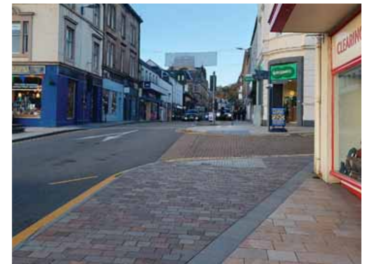
Looking north from George Street adjacent to the junction of A85. Good quality surface and the only crossing point with tactile can be seen at the southern point.
