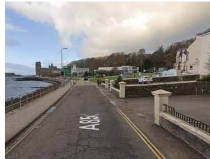
Image 2 | View north on Corran Esplanade at northern pinch point extent, adjacent to the Great Western Hotel.
