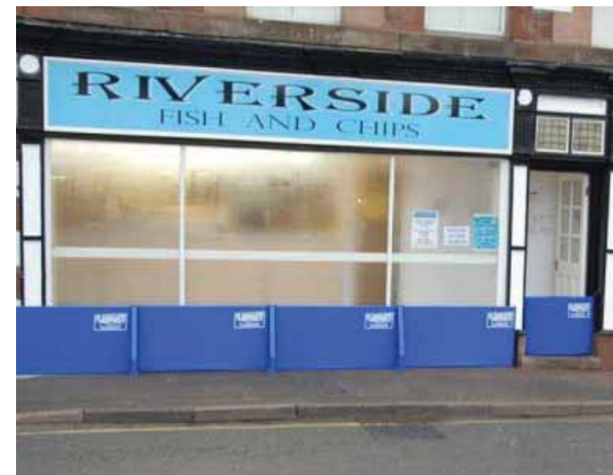
Example of Demountable Property Level Protection Image Source: Oban Flood Study Community Feedback Event Presentation (June 2019)
