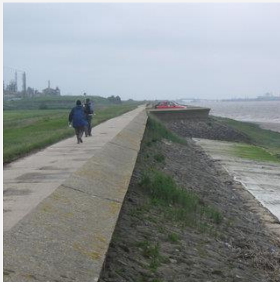
Embankment (Multi-functional space)
