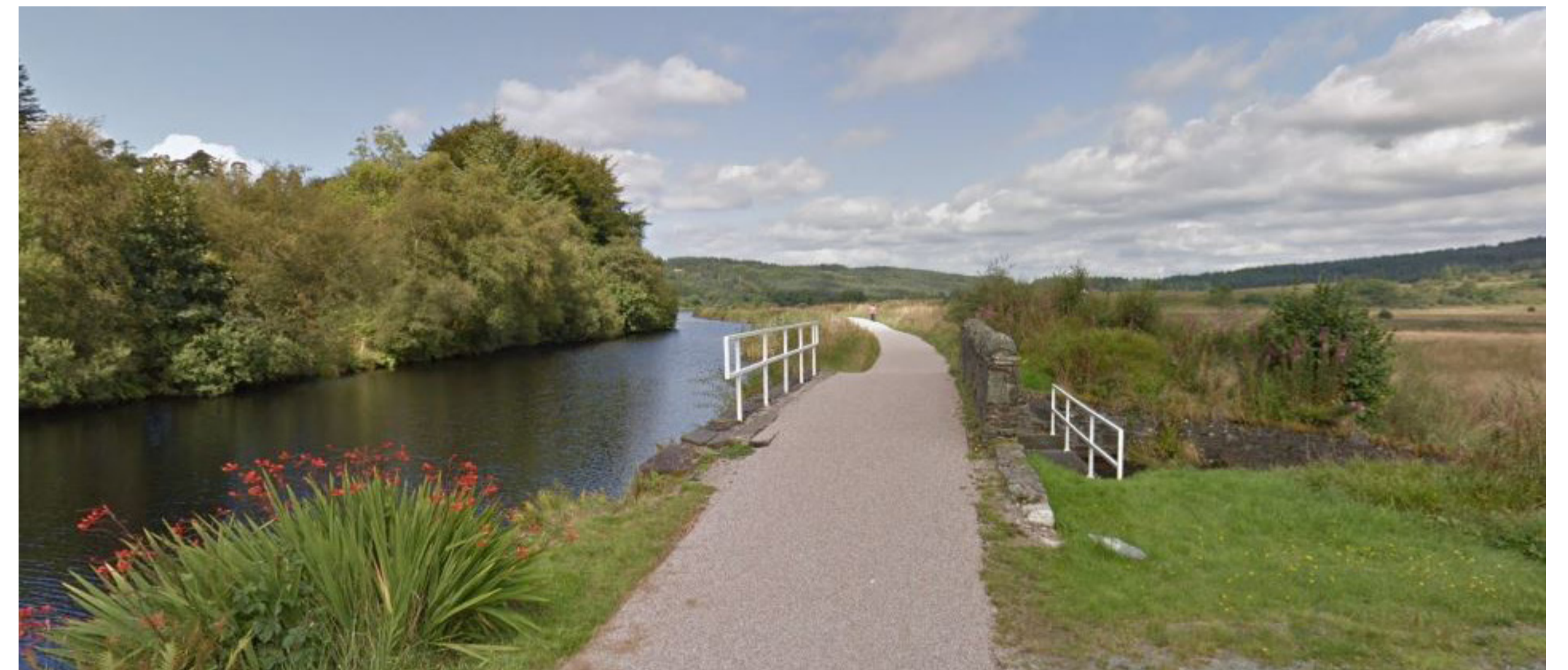
Change in operation of the Crinan Canal
