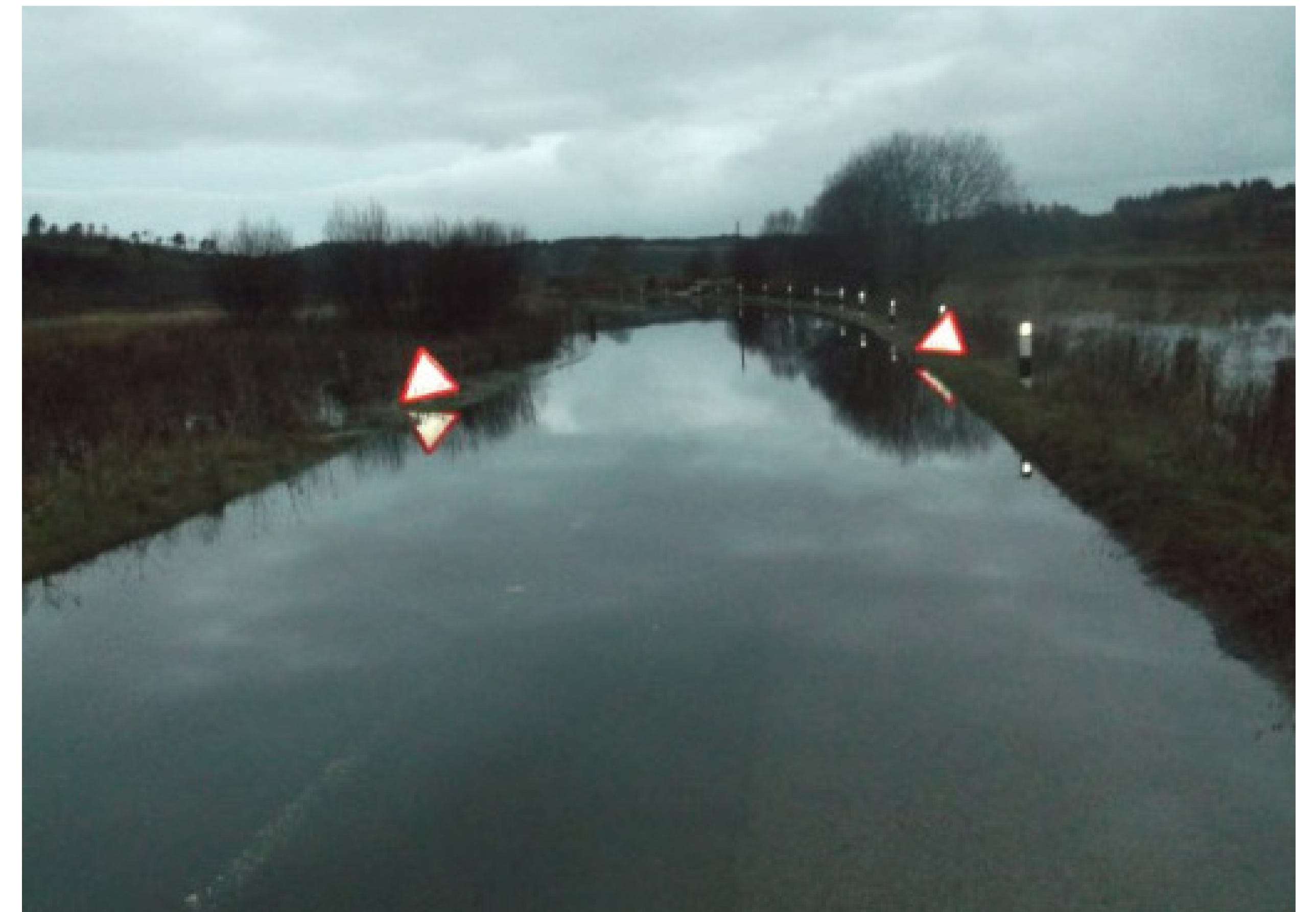
Flooding from the Badden Burn on the A816, north of Lochgilphead, 2014
