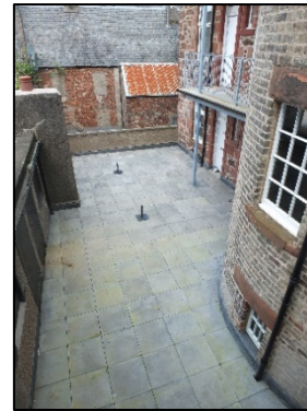
Rear deck - After
