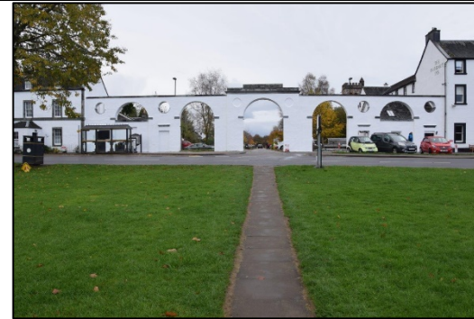
After work completed
