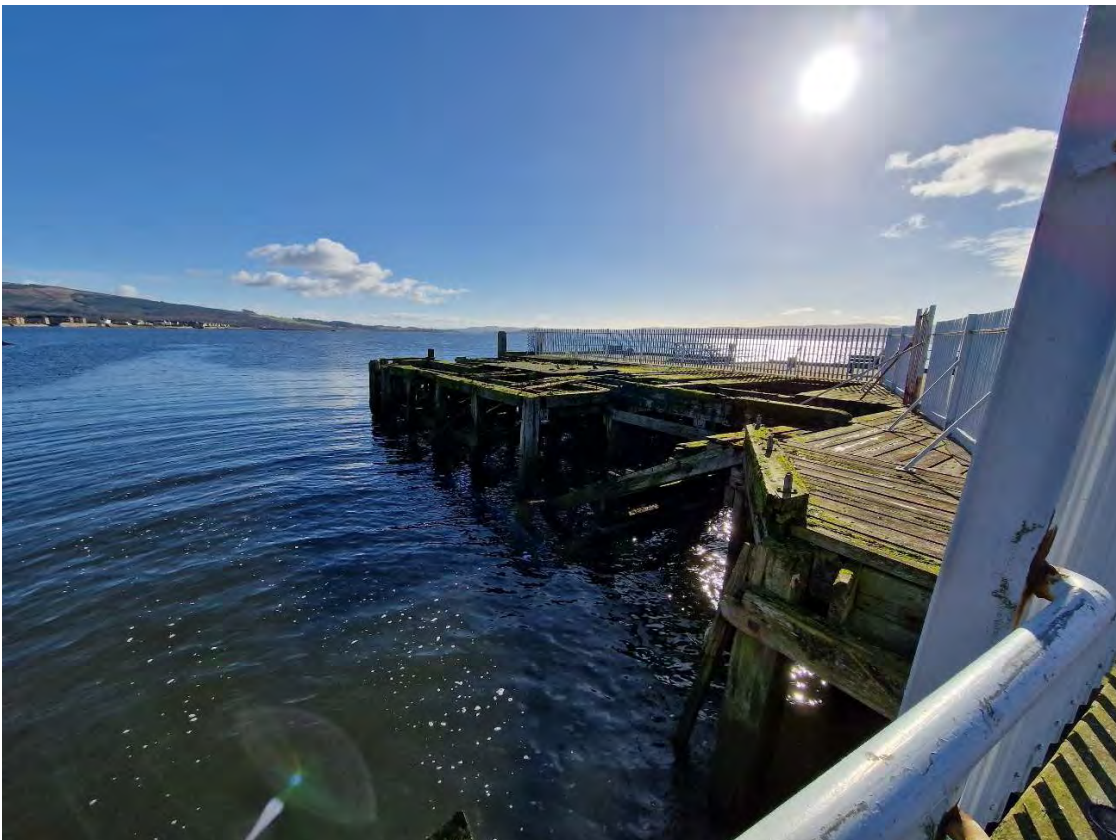
Figure App B 8: Fire Damaged Section of Pierhead (1)
