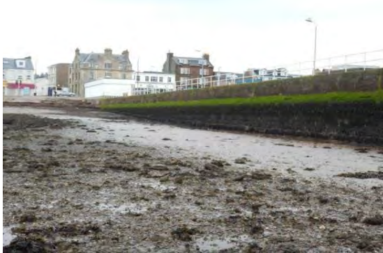
Showing north west face of masonry pier
