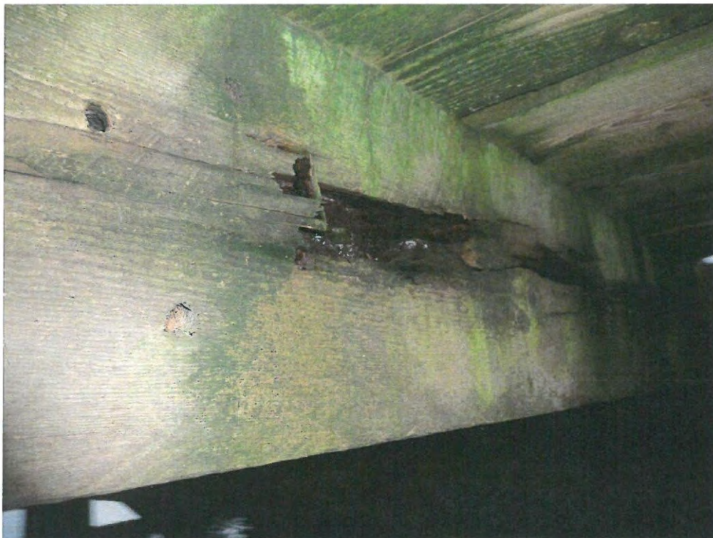
Photograph 14 Example of a softwood deck joist significantly decayed.
