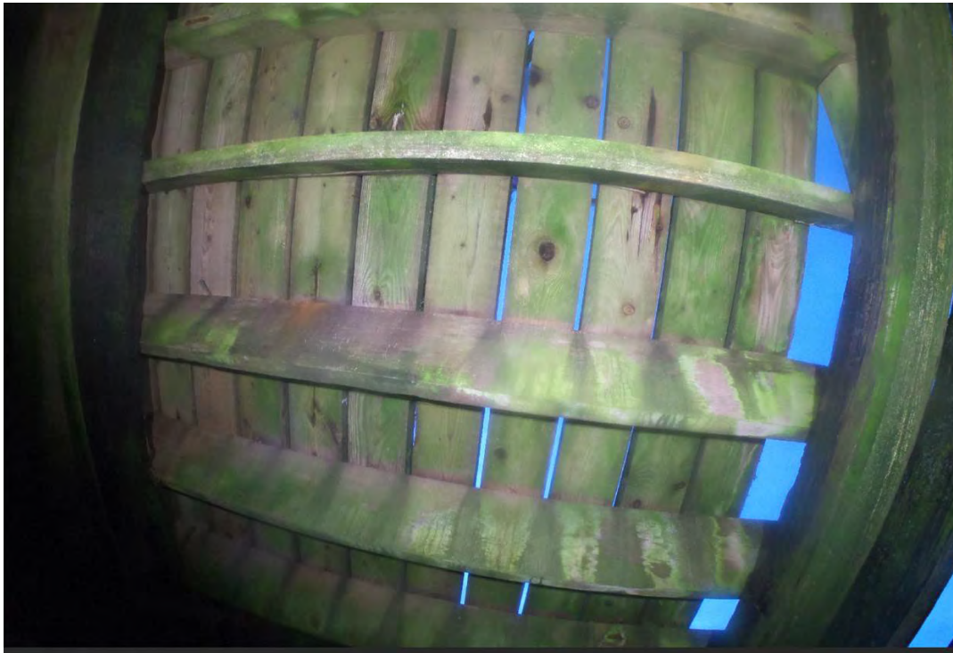
FIGURE 20: Helensburgh Pier – Angled rafters (“G” in Figure 19)
