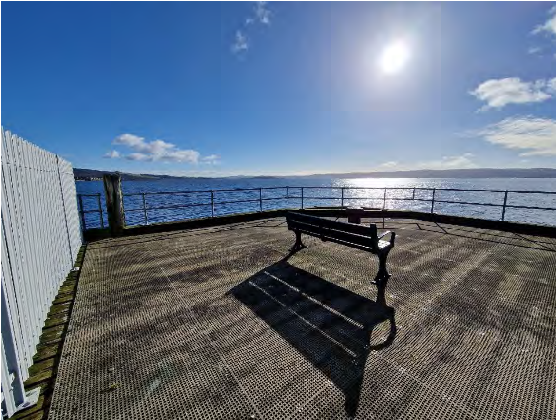
Figure App B 11: South-East Corner of Pierhead
