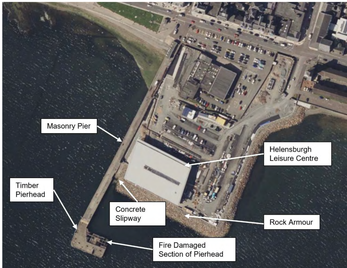
Figure 4.1 Helensburgh Pier Overview
