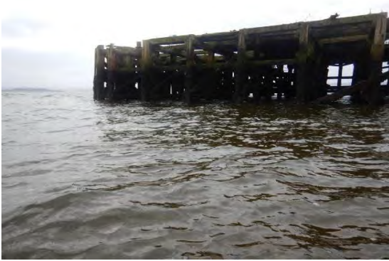
Showing north east face of timber pier
