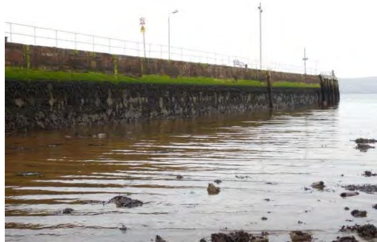
Showing southern face of masonry pier
