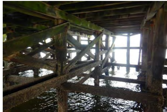
Showing construction below deck
