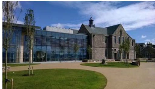
Accessible entrance at front of building
