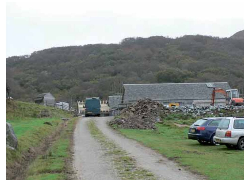
NK5 - Existing buildings and extensions under construction
