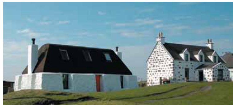
good quality refurbishment; distinctive proportions and strong simple shape retained
