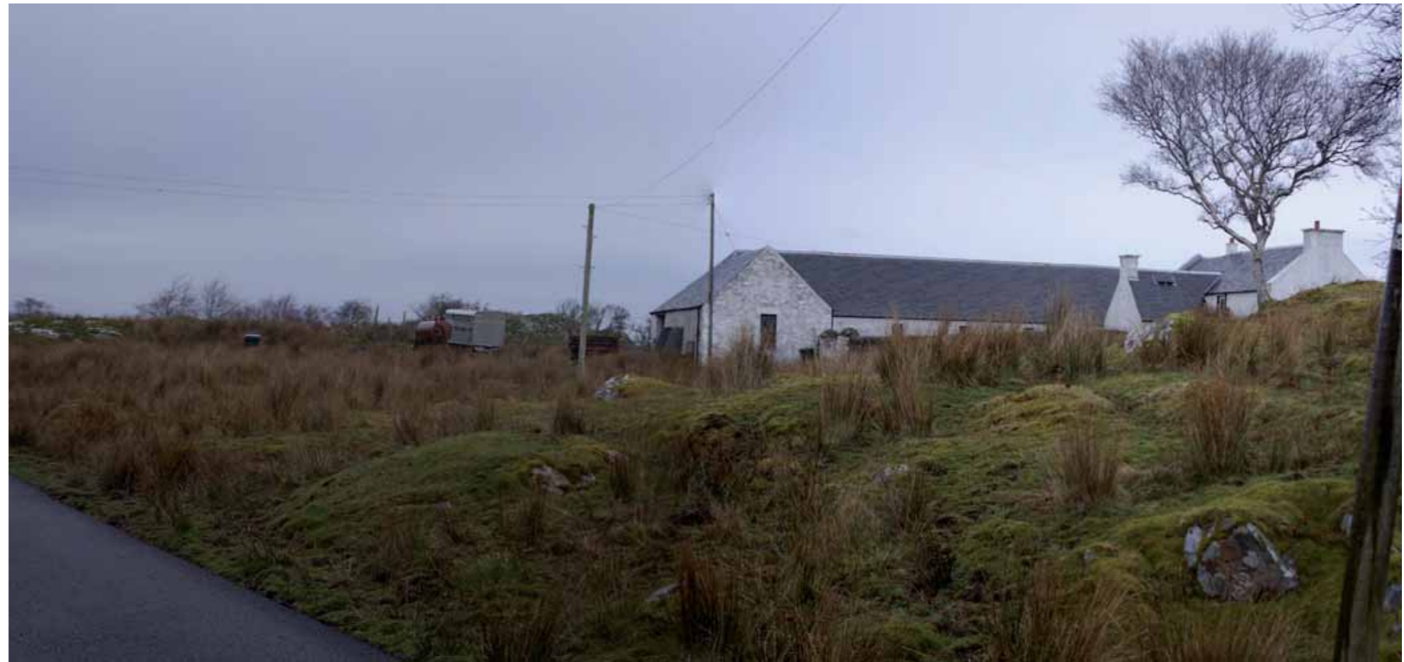
IS2 - looking northeast from road to Trudernish Farm
