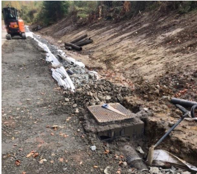
Construction of widened carriageway section and filter drainage, linked to existing culverts
