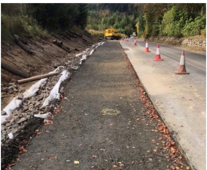
Widened North Bound lane and drainage
