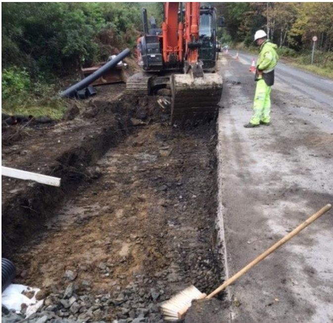
Construction of widened carriageway section and filter drainage, linked to existing culverts
