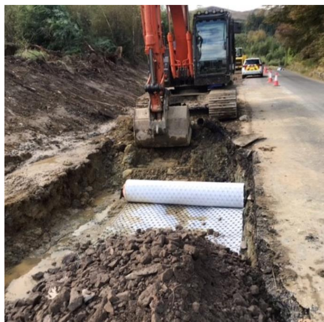
Construction of widened carriageway section and filter drainage, linked to existing culverts
