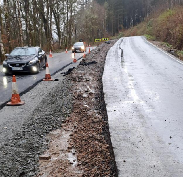
Reduction in vertical alignment and widening to 2 lanes 6.5 m minimum
