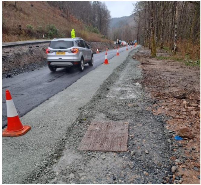
Reduction in vertical alignment and widening to 2 lanes 6.5 m minimum
