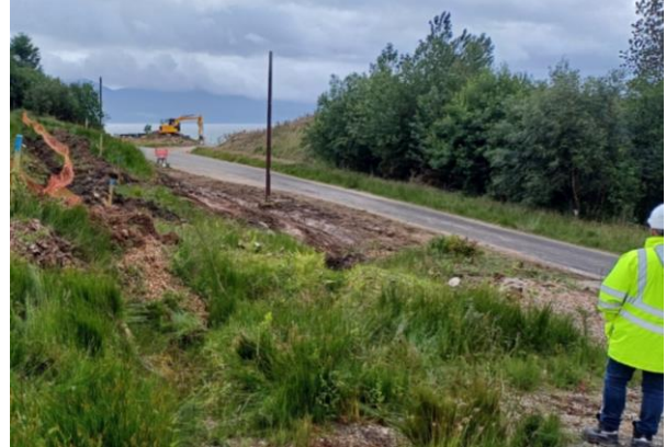
Initial excavation and removal of unsuitable.
