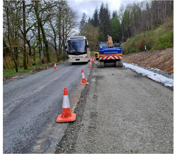
Reduction in vertical alignment and widening to 2 lanes 6.5 m minimum
