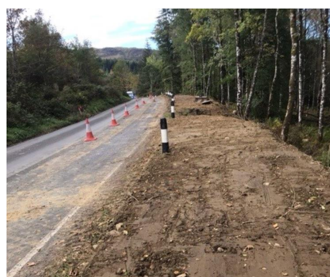
Enhanced Southbound embankment
