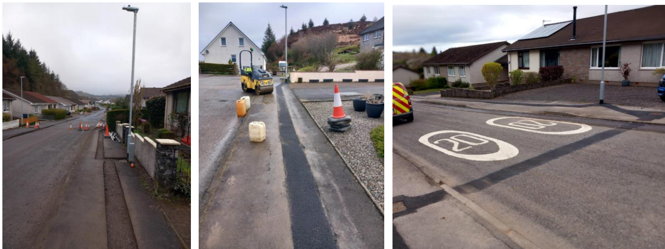
Nant Drive – Oban, Street Lighting duct, cable and column replacement.
