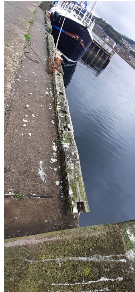
Image B4. Campbeltown, Old Quay wooden edge beams
