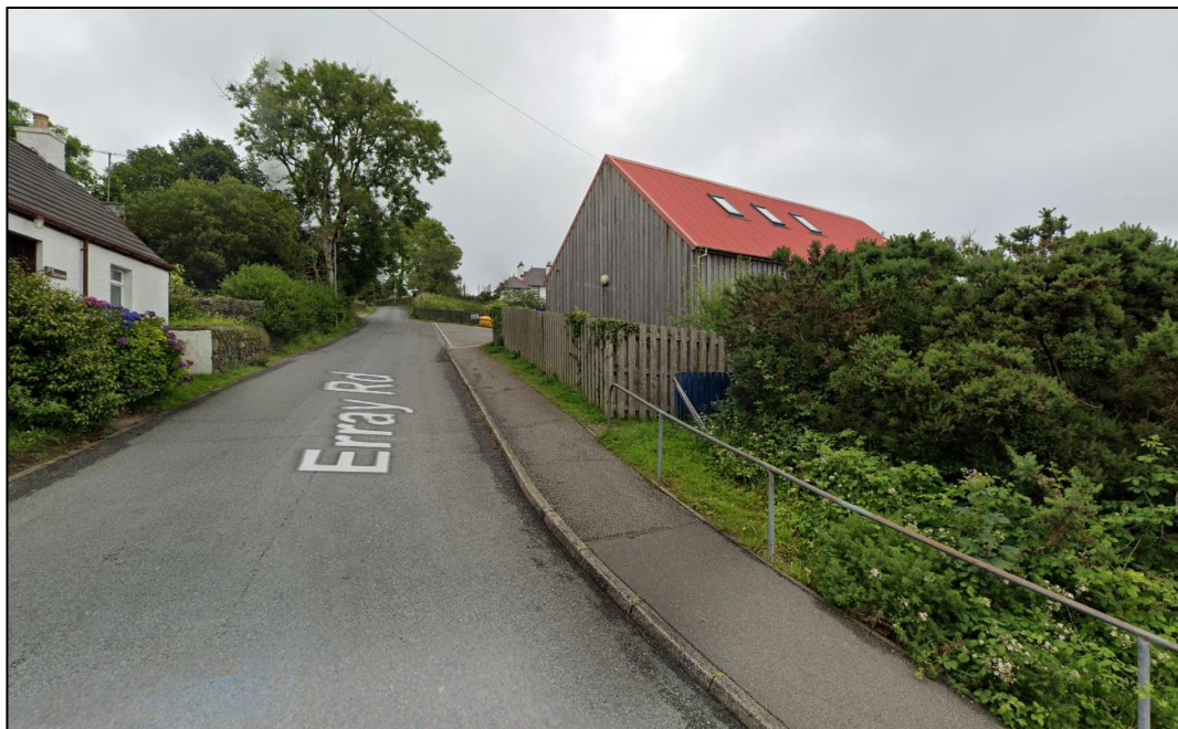
Figure 4. Footways on Erray Road
