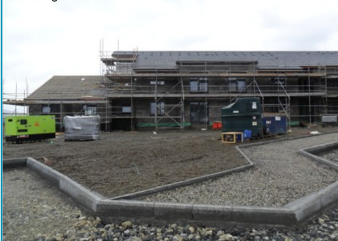
Mull Progressive Care Centre under construction
