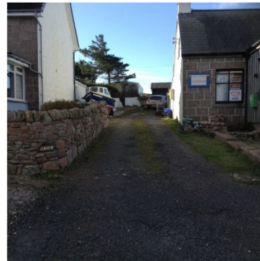
View of building from driveway
