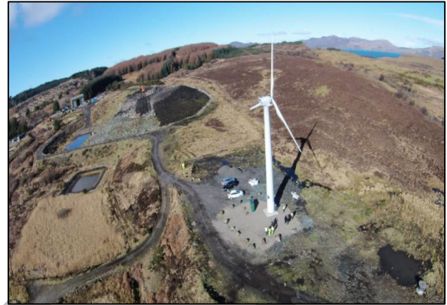
Council owned wind turbine @ Glengorm Landfill, Mull
