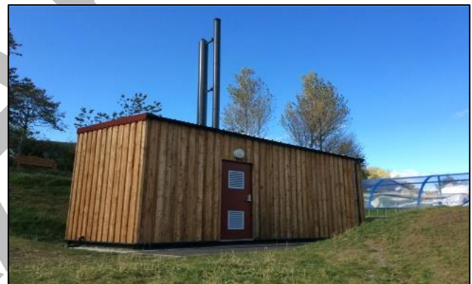
Ardrishaig Primary School biomass boilerhouse
