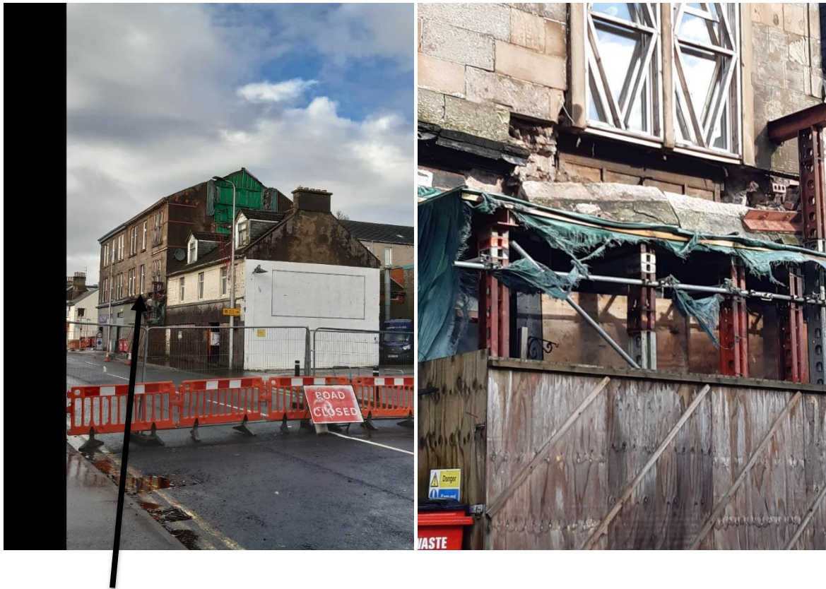
5-7 East Clyde Street- affected building
