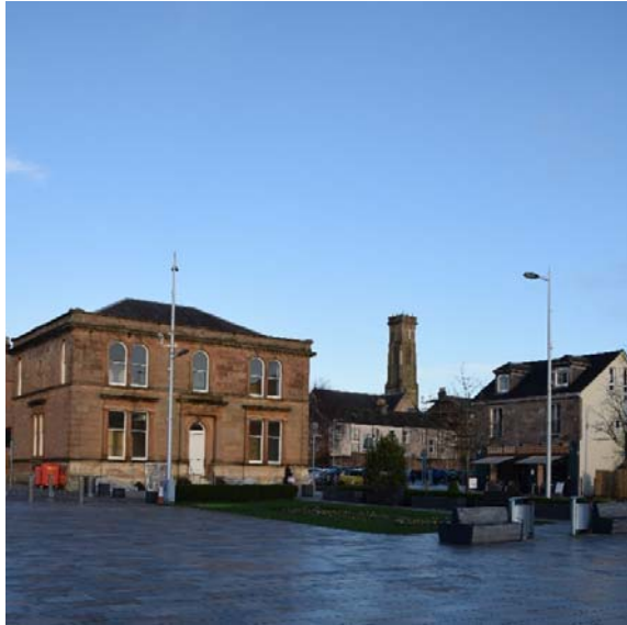
Open internal corner to north east side of Colquhoun Square. This affords long distance views towards tower of former St Columba Church.
