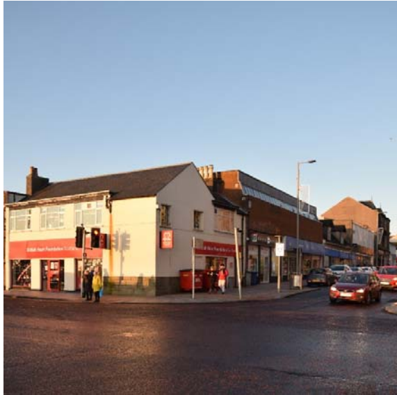
2-5 West Clyde Street to the corner of Sinclair Street and the adjoining building at 7-13 Sinclair Street are prime candidates for future redevelopment considering the long term enhancement of Helensburgh.
