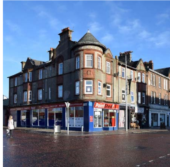
A L-shape three-story tenement at 74-78 of grey harl with red sandstone dressings with a squat turreted corner providing a robust termination to the end of the Town Centre area.
