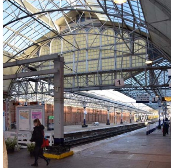
Helensburgh Central with its barrel-vaulted and pitched roof glazed canopies to platforms.
