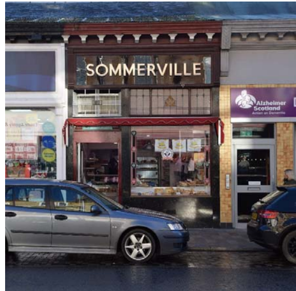
Late 19 th C, traditional shopfront to 21 West Princes Street. Mostly original with some later modern additions. Part of bungalow terrace row of shops. Shops either side have been replaced with modern designs.
