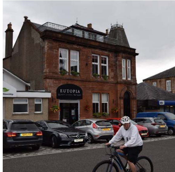
North side of Colquhoun Street. The single storey extensions affect the setting of the traditional buildings and are not positive in terms of streetscape.
