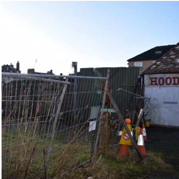
Ad hoc Heras fencing separating adjoining areas.
