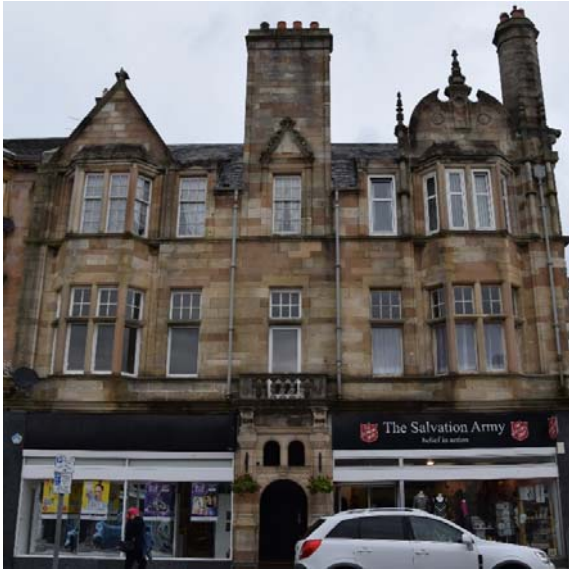
8-12 West Princes Street. A good example of traditional timber sash and case windows and a demonstration of their importance to the overall building character, in this case Jacobean with its original 6 over 6 and 6 over 1 glazing patterns formed with astragals. One flat has replacement modern Upvc casements which have a vastly different aesthetic with larger, double frames due to being a casement type. This begins to alter the character of the listed building.
