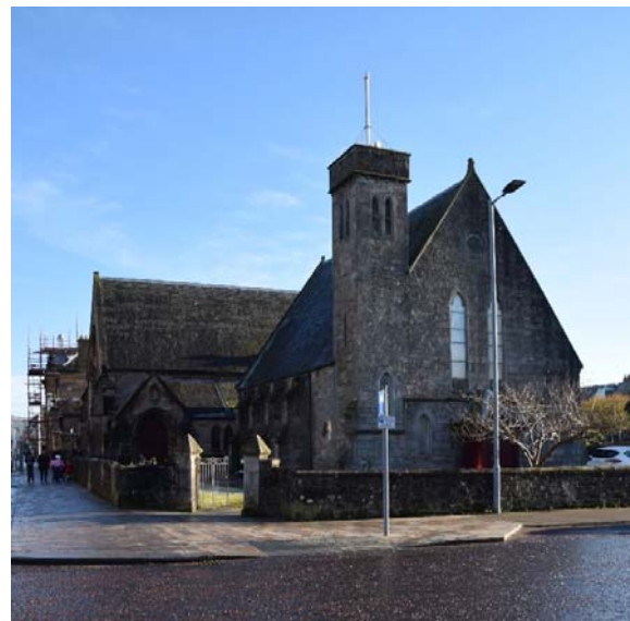
Helensburgh URC Church at the corner of Princes and James Street. The boundary wall is important in providing enclosure to the church grounds and maintaining the consistency of urban block reinforcing the grid iron street pattern.
