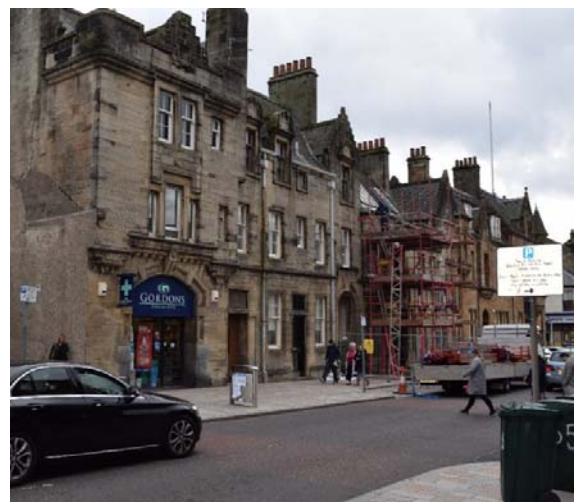
48-52a Sinclair Street. A N Paterson's 1906 addition originally comprising the Police Office and Fire Station. Continuing the Scots vocabulary of the former Town hall but with a modern interpretation
