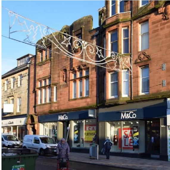
38-40 Sinclair Street. Former Helensburgh and Gareloch Conservative Club. Elegant asymmetric elevation with highly distinctive parapet and exquisite carved masonry.
