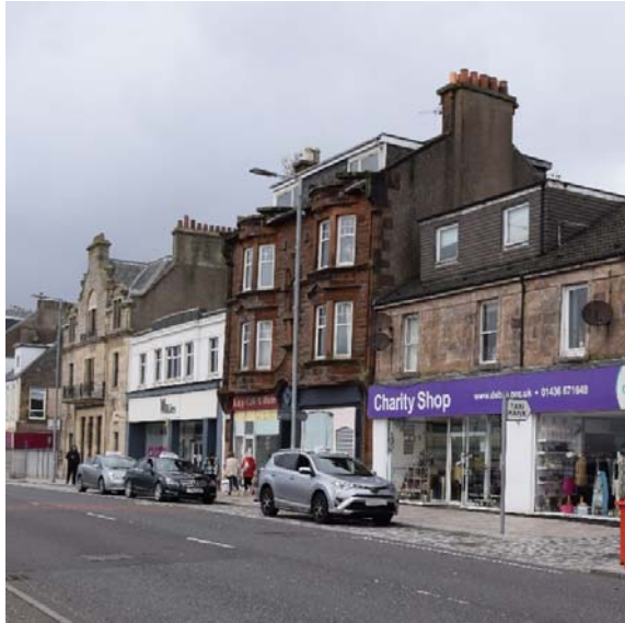
18 West Clyde Street. T and J Low. 1909. 3 Bay Glasgow style tenement with dated keystone, full height bowed tripartite oriels flanking and corbelled stepped bowed parapet with breaking eaves.
