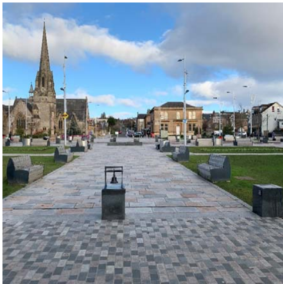
Public realm works to Colquhoun Square.
