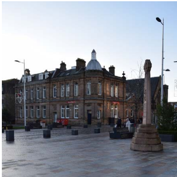
18 Colquhoun Square, W W Robertson, 1861. Late Victorian former post office with elongated cupola provides a strong corner feature and prominent visual marker.
