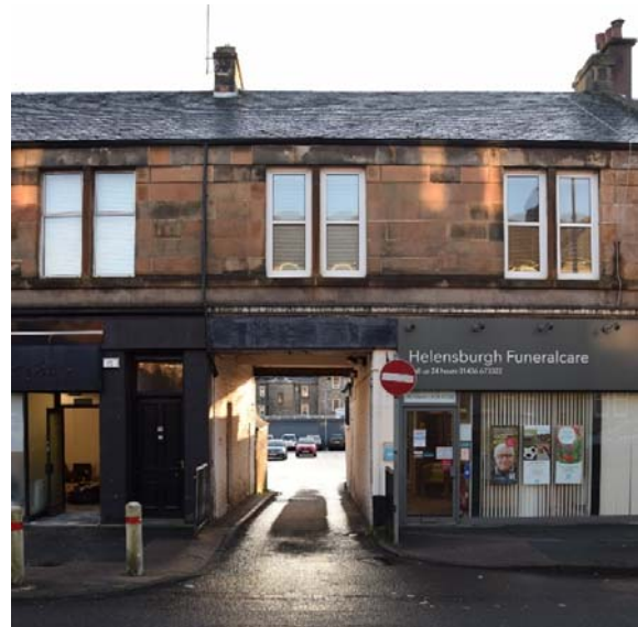
Pend to King Street forming the exit to the principal car park behind.
