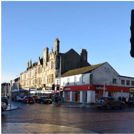
8-12 West Princes Street. Striking tenement in Jacobean style with its varied skyline and prominent chimney stacks. The building has an impressive scale on Princes Street and makes a significant contribution to the street scape. Adjoining to the west is William Tait's well-proportioned tenement.
