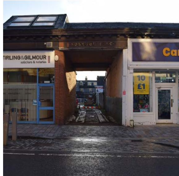
Pend to West Princes Street as part of bungalow row of shops. The rear courts are visible from the street and their appearance directly affects the character of the town centre. Consideration should be given to how these are used.
