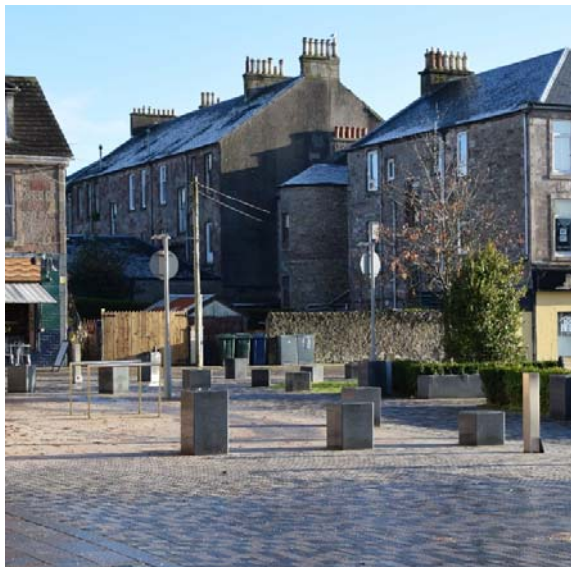
North east side of Colquhoun Square. Gaps in frontages offering views into interior spaces of the block and rear facing elevations.
