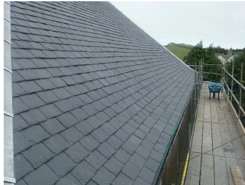
New roof at Smith Drive, Campbeltown
