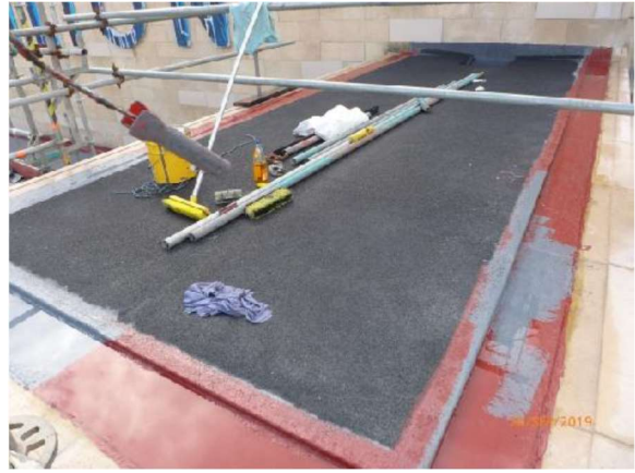
General View: over Stair 2.
