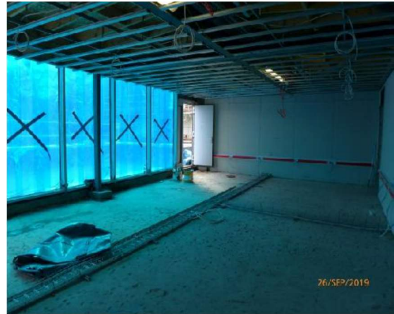
New Offices: General view of middle office.
