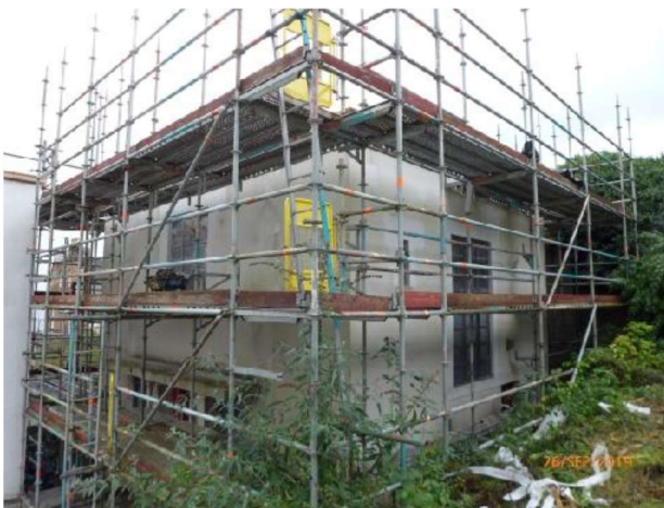
West & South Elevations – Caretakers House (NB: new windows in situ).
