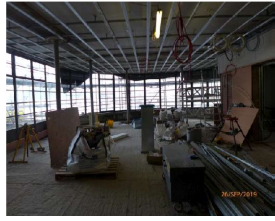
Looking East: general view of Café Area.
