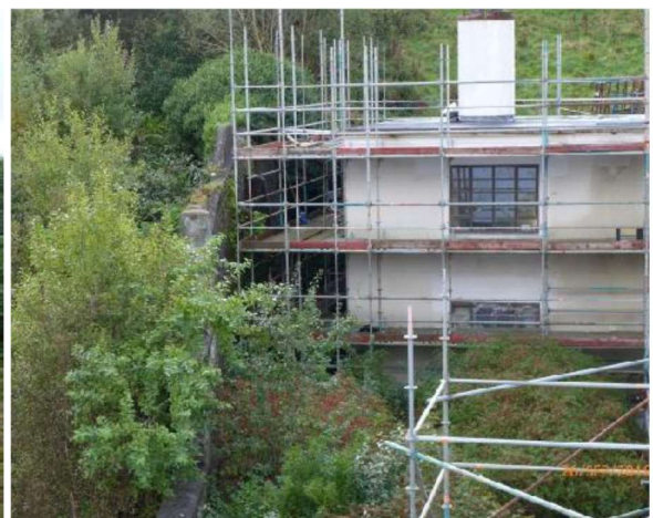
East Elevation – Caretakers House.
