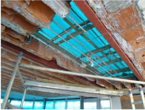
General View - Sections of the existing roof slab broken out to form the opening for the new AOV.
