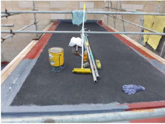
General View: over Stair 2.
