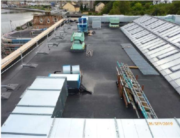
General views: Main Hall Rooflight – east facing area looking south.
