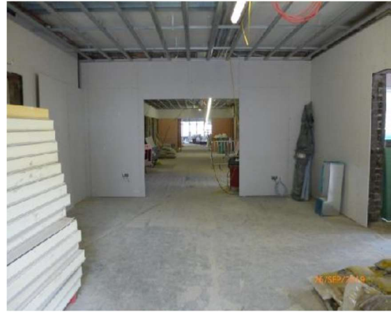
Looking East: General view of Multipurpose Flexible space area.
