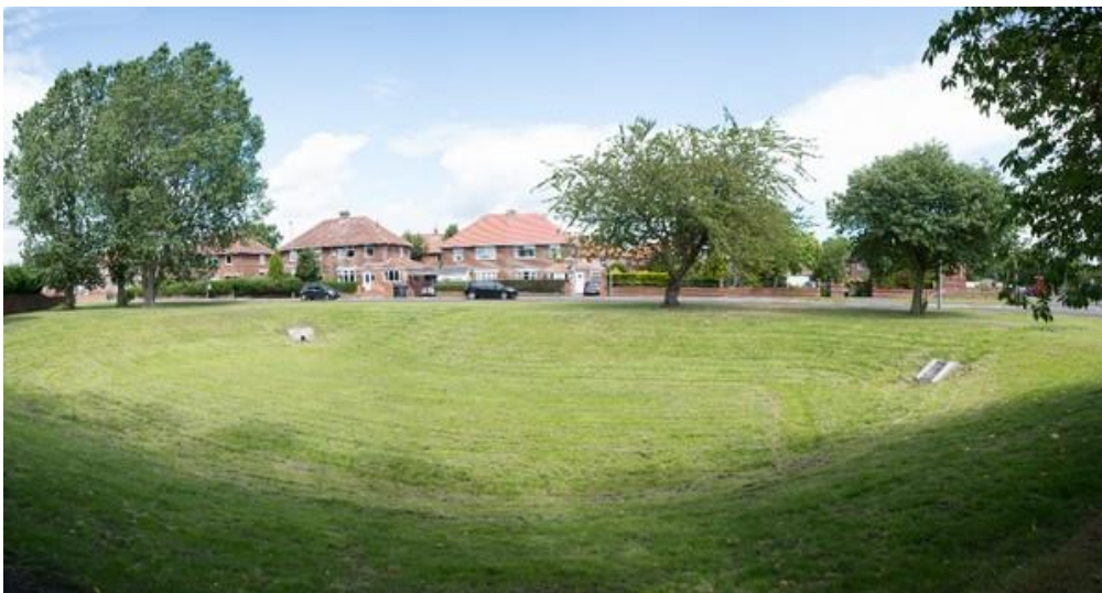
Figure 3-2 Typical detention basin
