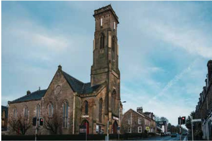
The Tower Digital Arts Centre
