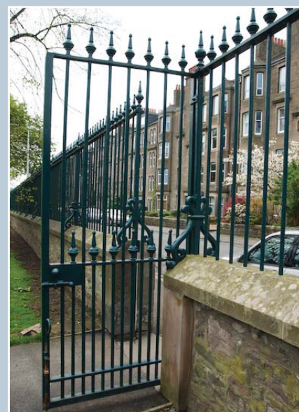
Railings reinstated in 2006 define the edge of Baxter Park, Dundee, and are key to its regeneration and good management. The patterns were deduced from a short surviving section.
