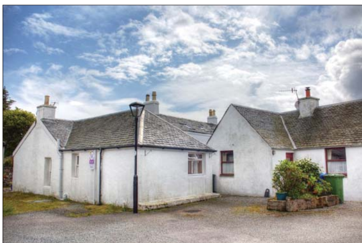
Hipped end of newer extension
