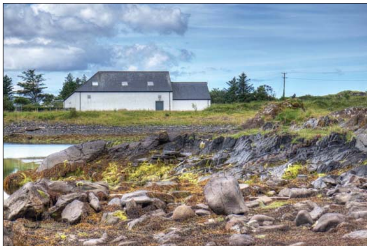
The Community Centre, showing hipped roof
