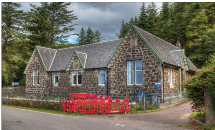
The School—note: repairs have subsequently been carried out to the boundary wall
