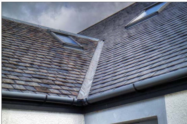
New and reclaimed slates on Community Centre
