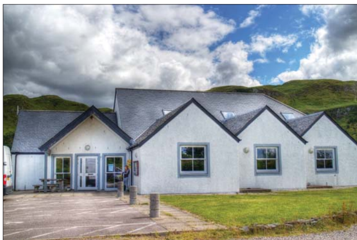
The Community Centre, showing square windows and full length sash and case windows
