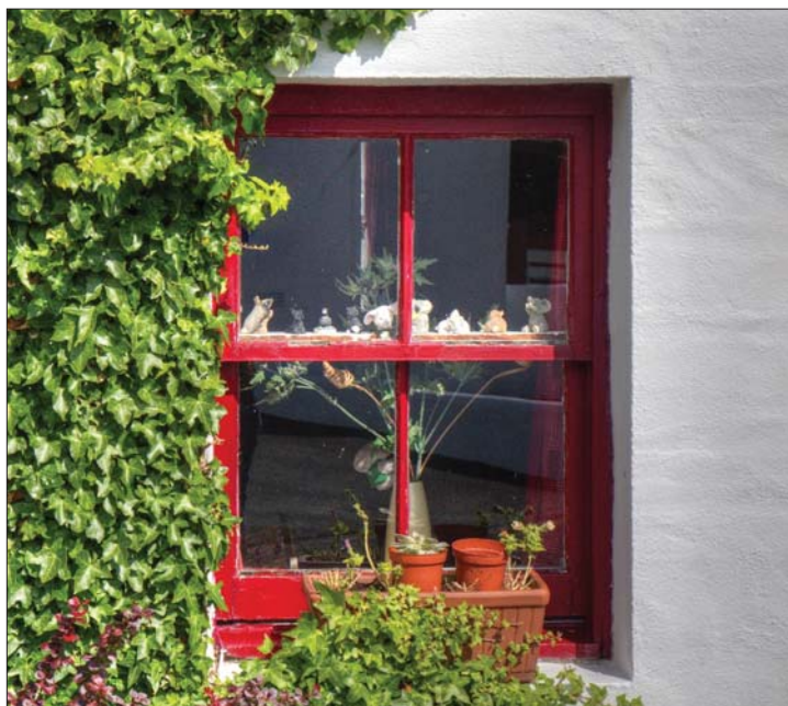
Traditional sash and case window with slim astragals
