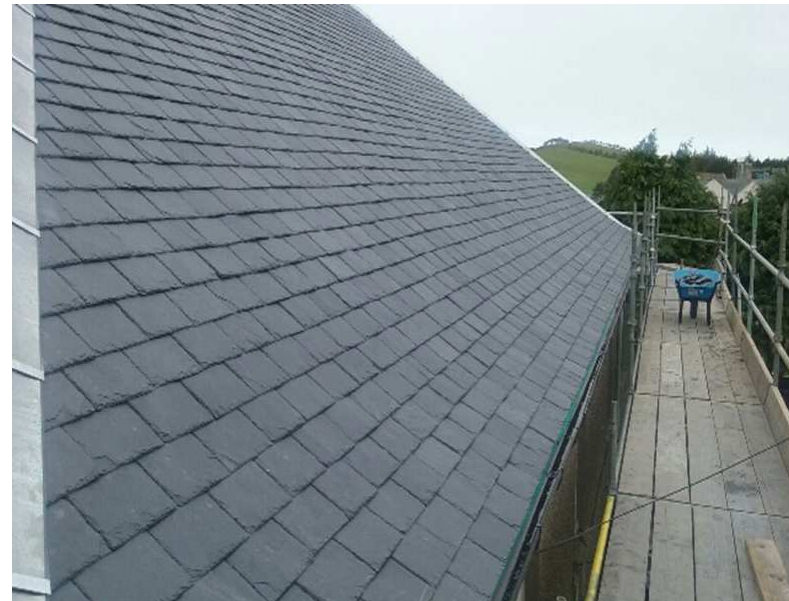
New roof at Smith Drive, Campbeltown
