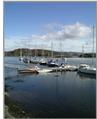
Floating pontoons for recreational sailing and power vessels in Tarbert Harbour
