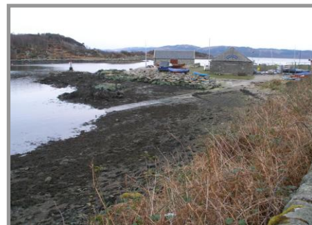
Tarbert Sailing Club and slipway with fish processing facility in the background
