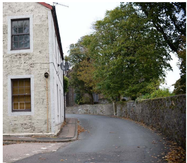
Boundary wall 3. The category B Listed wall to Castle Gardens
