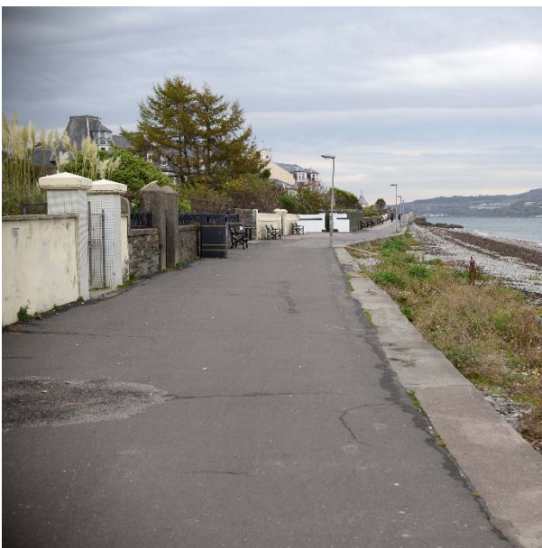
Photograph of Victoria Parade illustrating the key role of the boundary condition in defining the character of shore frontage and promenade.
