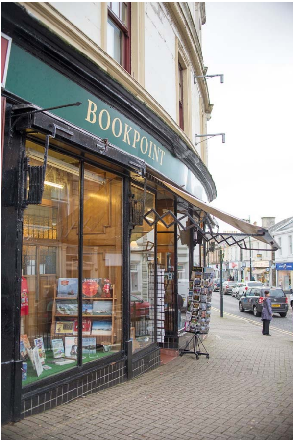
The curved shopfronts to Ferry Brae
