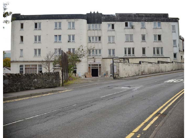
McColl's Hotel – prior to demolition
