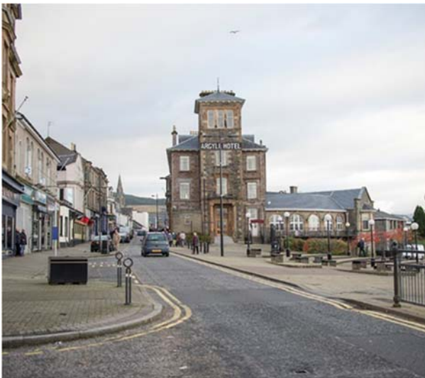
The Argyll Hotel. Began mid 19 th Century. The hotel is a key landmark building with the campanile-like tower a strong townscape feature. The bandstand area, created after reclamation to connect the esplanade to East bay is key to the setting of the building.
