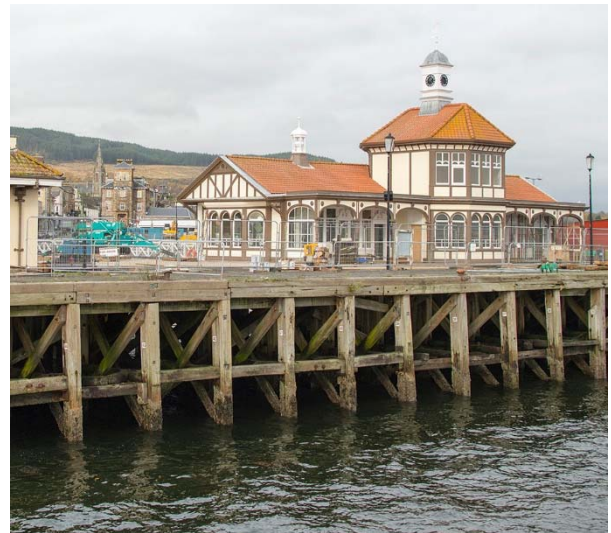
Waiting Room and Pier Masters Office from the quayside. Dunoon Pier - Clarke and Bell with Sir William Copland in collaboration with R A Brydon and C J M Mackintosh, 1896-98; incorporating earlier pier to N by Campbell Douglas, 1867-68 Largely retaining its original form and distinctive detailing, it is acknowledged as the finest Victorian pier building of its type in the country. It is of crucial importance to the Dunoon's historic character
