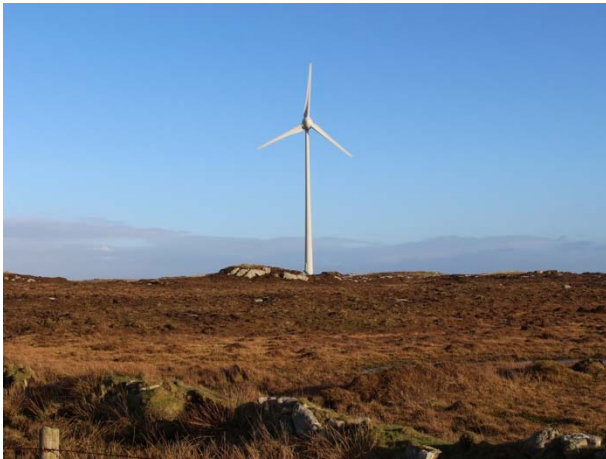
Existing community wind turbine located in the north-eastern part of this LCT
